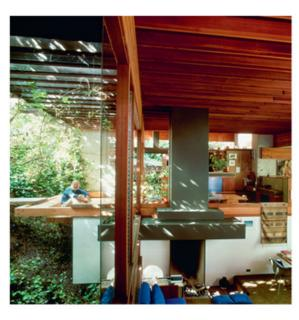
Ray Kappe sits on the deck of the house he built for his family. Six concrete towers support laminated redwood beams that enclose a multilevel interior.
