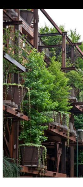
Widely known grean wall schemes wouldn't have worked in the case, because they require a vertical surface for the plants to be properly watered and ted. Instead, the project uses a bespelor facade system, in which standard rectangutar planters are mounted on a supertructure made or metal tubes and rate, with spocally developed joints that allow creating the developed institual shape.
