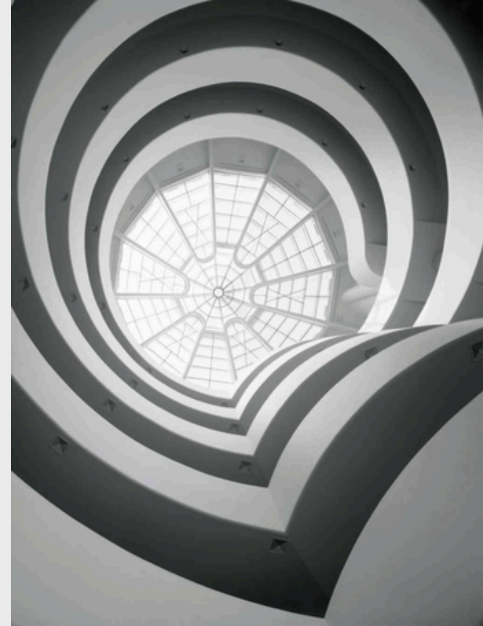
15 Solomon R. Guggenheim Museum, New York (1943–59), designed by Frank Lloyd Wright. Artworks are displayed on the outer walls of the upwardly spiralling concrete ramp.
