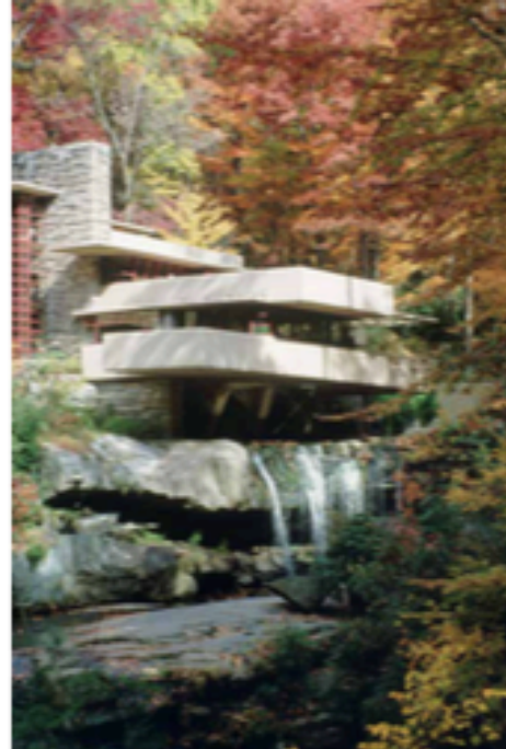
16 Frank Lloyd Wright's greatest 'natural' house: Fallingwater (1938), Mill Run, Pennsylvania. Anchored to the rock by solid masonry walls, the reinforced-concrete floors and ceilings cantilever out over the waterfall.
